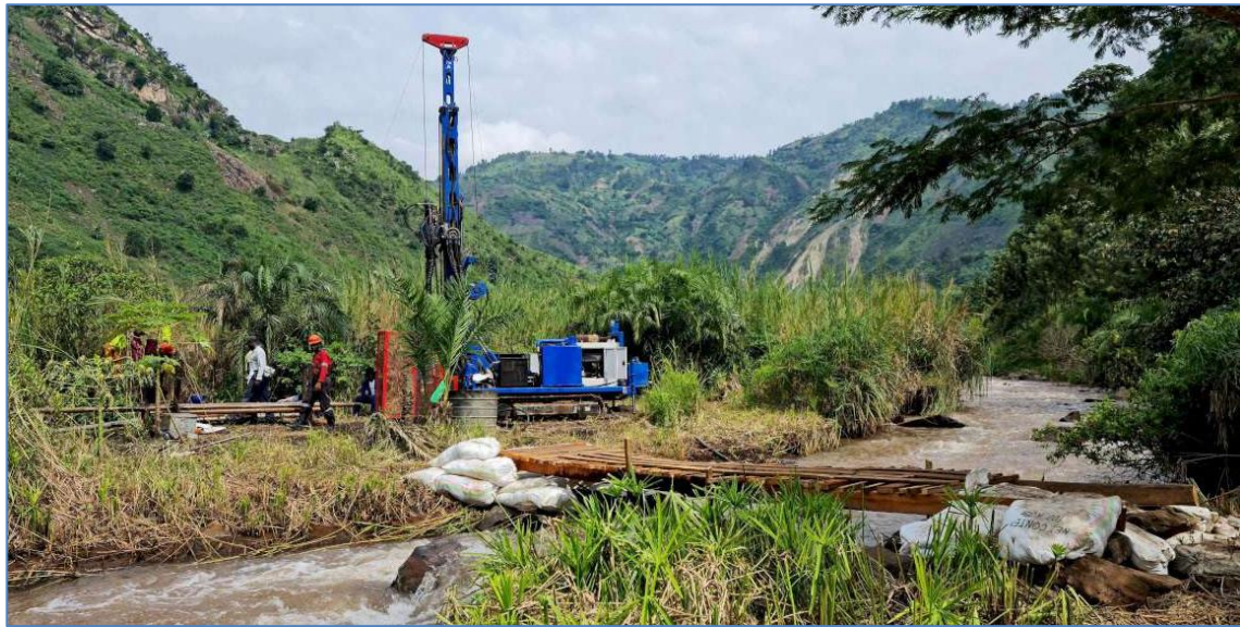
Figure 3-1 – Borehole Drilling During Geotechnical Studies
